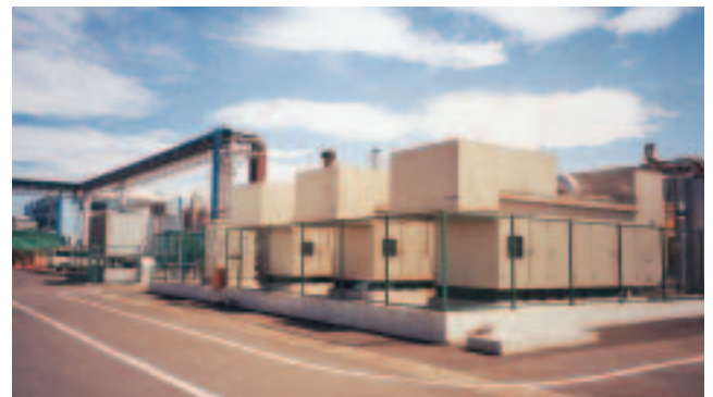
Cogeneration system (Kawagoe Plant)
